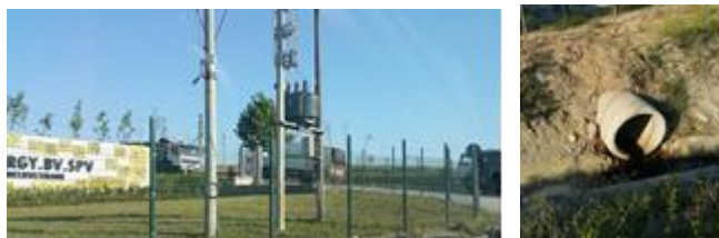
Fig.3 Discharge of Sharra's landfill wastewater into the river [Photo: Mariglen Kume]
