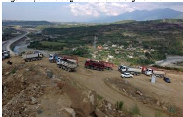
Fig.4 view of the highway Tirana-Elbasan works
